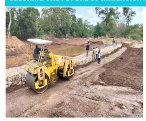
At **TARDA**, we are taking bold steps to protect and enhance the Tana Delta Irrigation Project (TDIP). The ongoing Gabion Protection Works at Kelona Brook are a game-changer—fortifying riverbanks, preventing soil erosion, and ensuring stable water flow for irrigation.
