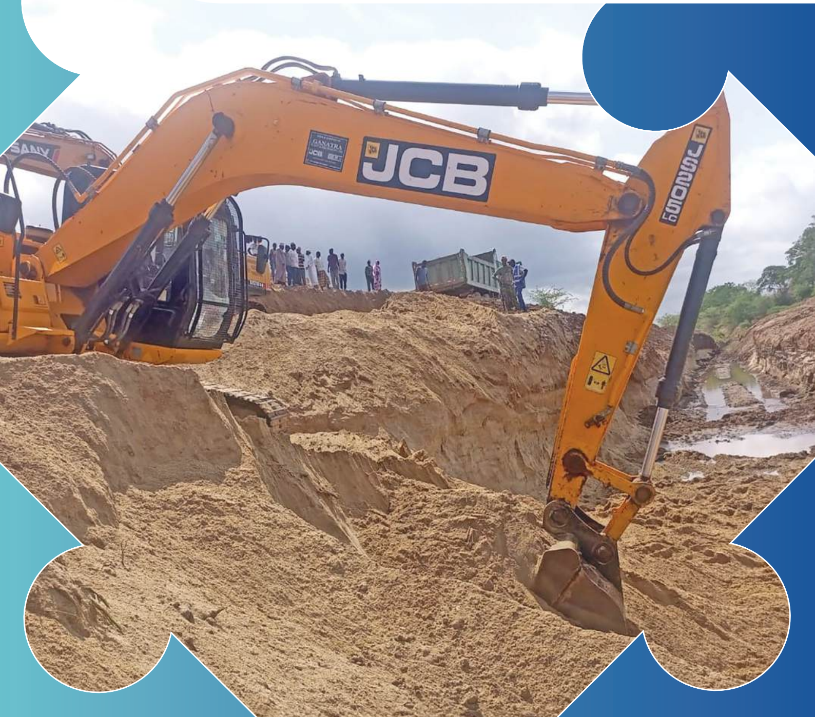
Rehabilitation of Kitere Water Intake at Tana Delta Irrigation Project
